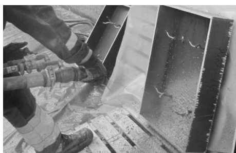
Fig. 4 Shot-creting of Höganäs Pump LC50
