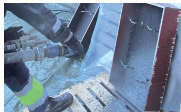
Fig. 4 Shot-creting of HÖGANÄS PUMP LC 50 AR
