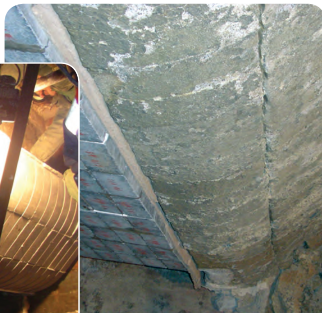
Bullnose blocks during Installation at Norcem's Brevik cement plant, Norway
