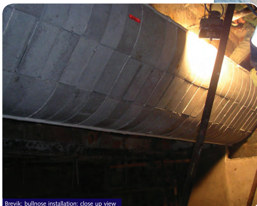
Brevik: bullnose installation: close up view
