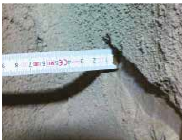
Figure 4. Lining after three campaigns, 2013.
